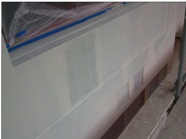
Detail Plaster and Bandaging applied to cracks
