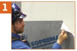
Peel off the top portion of the silicone release film and adhere the membrane to the substrate, making sure the membrane is well aligned.
