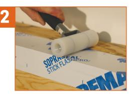
Adhere the bottom section by removing the silicone release film.\* Apply pressure using a roller to ensure maximum adhesion.
