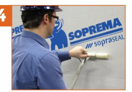
Use a roller to apply pressure over the entire surface of the membrane to ensure uniform adhesion to substrate.
