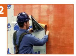
Peel off the top portion of the silicone release paper and adhere the membrane to the substrate, making sure the membrane is well aligned.
