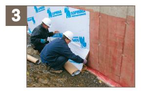
Gradually peel back the remaining silicone release film, making sure the membrane is completely adhered.
