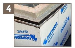
Use a Termination Bar and Alsan Mastic 2200 to seal details and critical areas. The use of an Equus approved protection and drainage board is recommended before backfilling to ensure the integrity of the waterproofing membrane.
