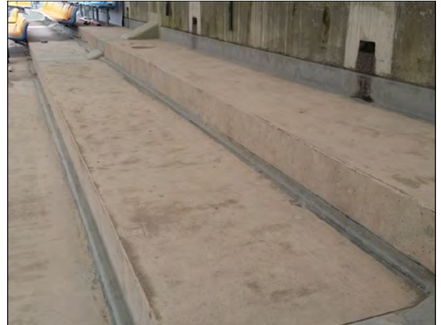
Prepared concrete substrate ready for application
