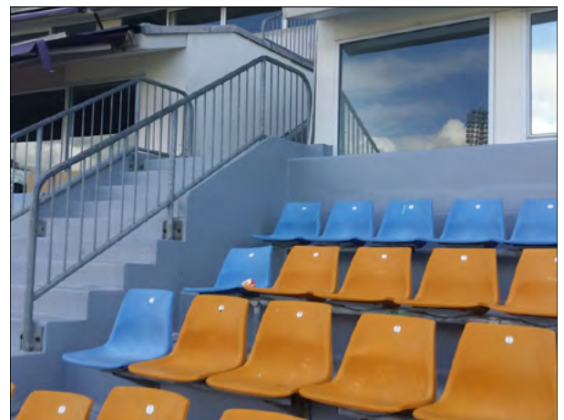
Matacyl Membrane applied to stairs and aisles
