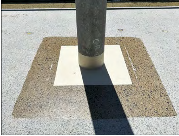
Area prepared and detailing coats installed
