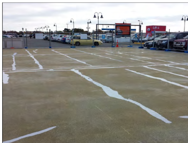
Crack repair to existing substrate
