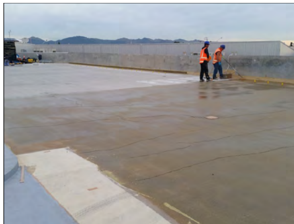
Primer Application to concrete substrate
