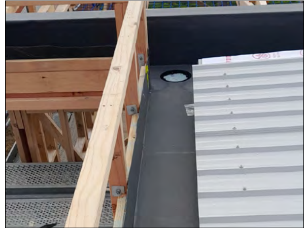
The FLAGON TPO 90 degrees external corners are in place for extra reinforcing and stability
