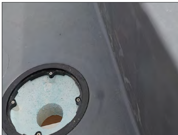
40mm welded TPO lap clamped tight into the outlet
