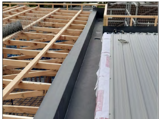
The FLAGON TPO membrane provides a smooth and aesthetical finish for internal gutters
