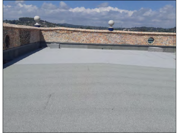
Warm roof completed after 2-layer Duo Landscape application
