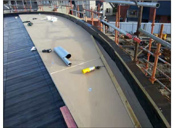
Installation of PIR Board over vapour barrier
