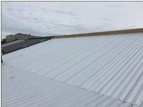
Metal substrate ready for warm roof installation
