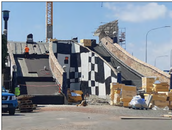
Ramp waterproofing underway
