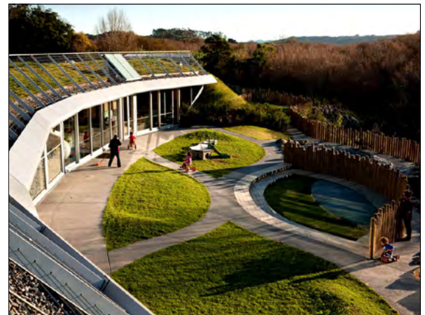
Finished project showing gutter edge
