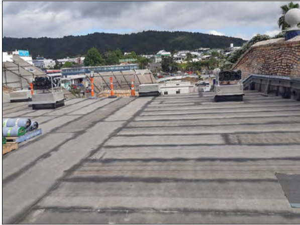
Vapour barrier installation
