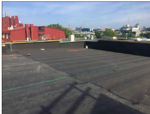
DeboTack Aero self adhesive basesheet applied over PIR thermal insulation board
