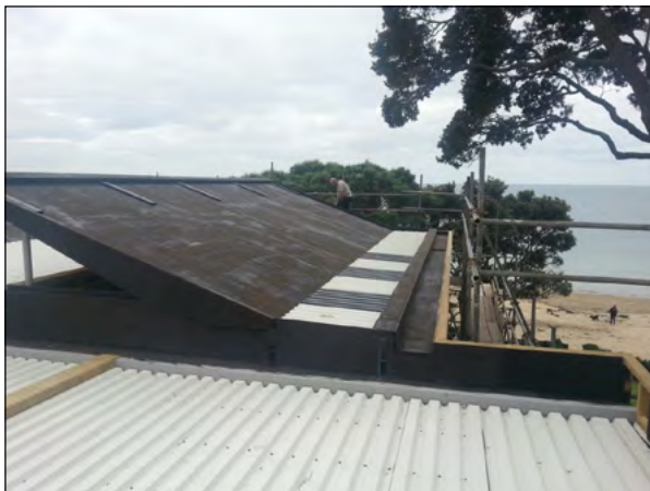
Substrate prepared for warm roof application
