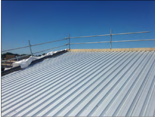
Metal tray roof ready for warm roof application
