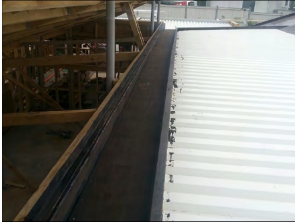
Metal substrate and primed gutters
