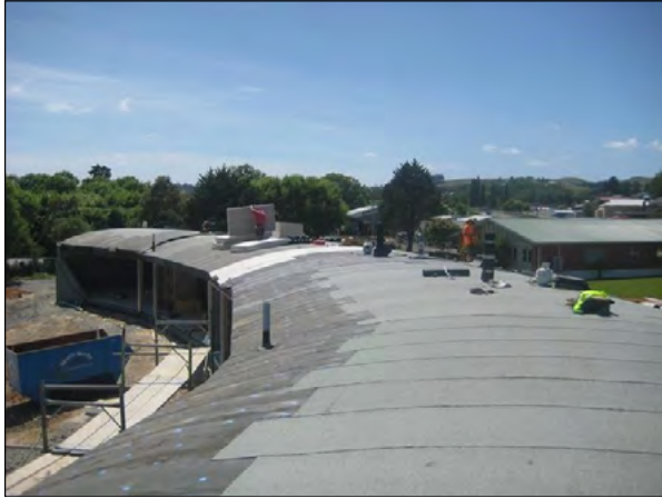
DuO capsheet installed over mechanically fastened basesheet and PIR thermal insulation board
