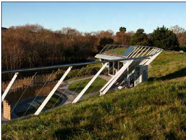
Green roof installed over DuO Landscape
