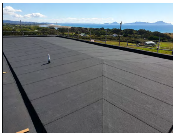
Finished DuO capsheet application
