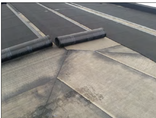
DuO AGR Capsheet installed over basesheet
