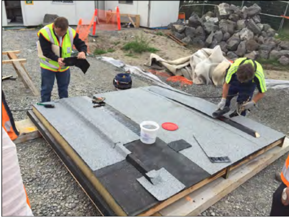
Preparation of the DuO mock roof
