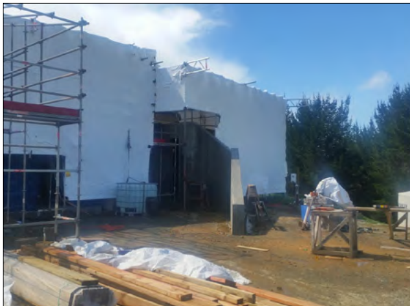
New build underway
