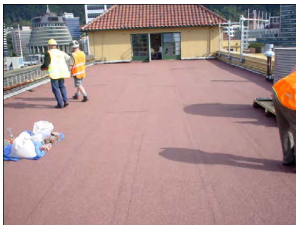
Completed roof refurbishment
