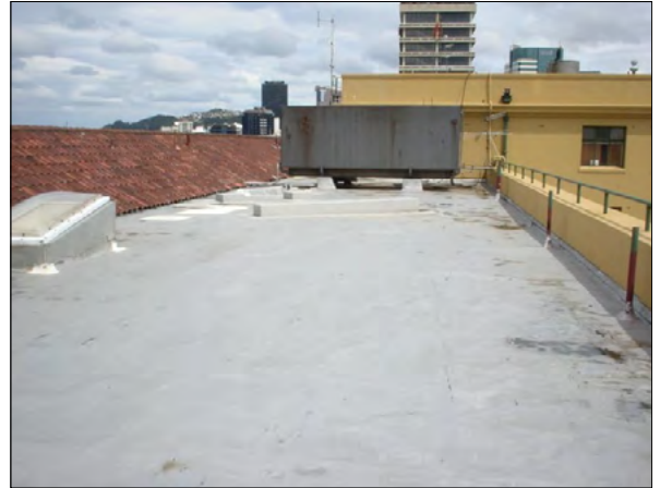
Existing roof before renovation
