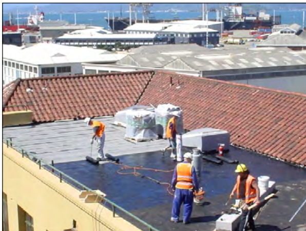
Preparation of area, primer and basesheet application
