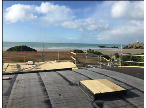
Installation of the DuO basesheet over plywood
