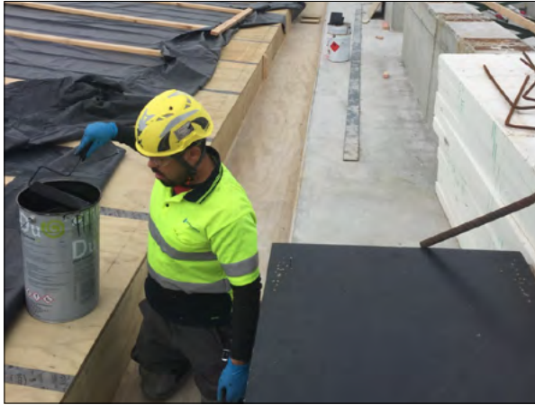
Primer application on plywood substrate
