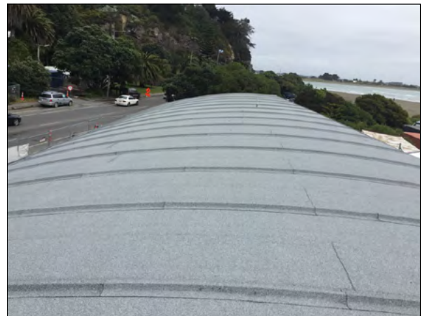
Finished top roof
