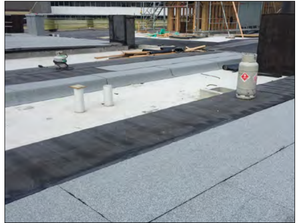
DuO Capsheet installation
