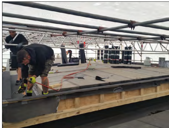
Deboplast Basesheet installed over plywood roof
