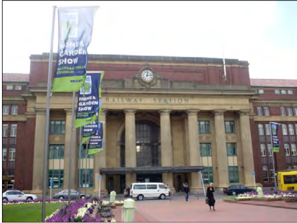
Wellington Railway Station Entrance
