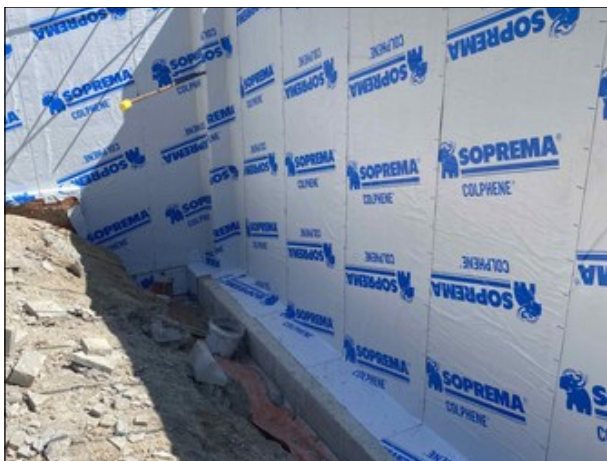
Completed wall waterproofing
