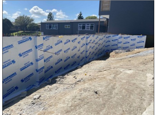
Installation of COLPHENE 3000 below-ground waterproofing
