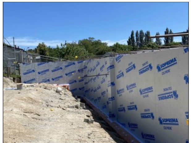
Connection of COLPHENE 3000 waterproofing membrane to DPM
