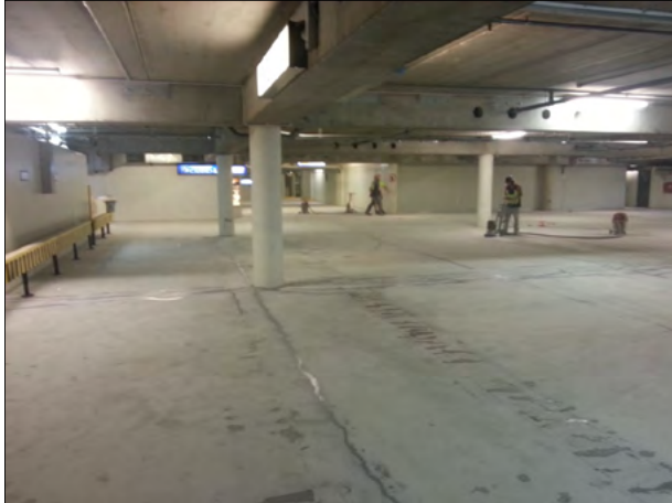
Concrete substrate preparation
