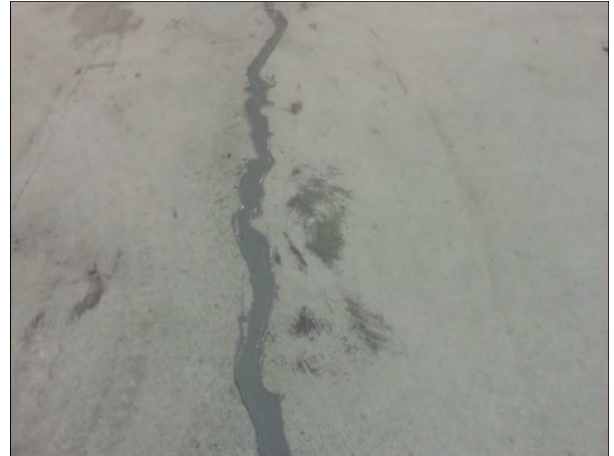
Crack repair with Sealboss crack injection
