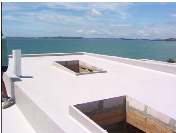
Dexx and fibreglass detailing around skylights
