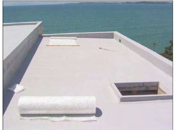
Fibreglass encapsulation into wet Dexx bodycoat
