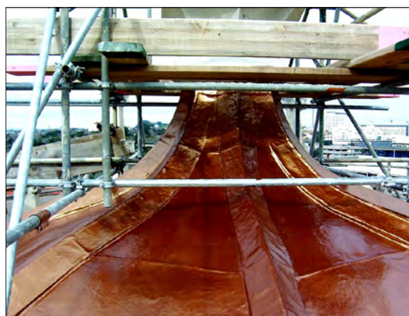
Chevaline Chemglaze protective clear finish applied
