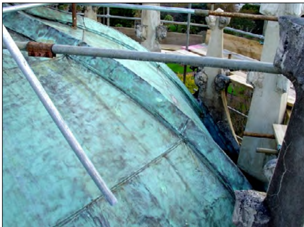
Original weathered copper roof
