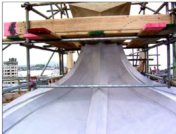
Chevaline DEXX base coat applied over copper
