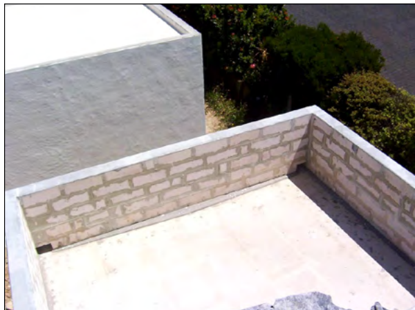
Hebel block structure
