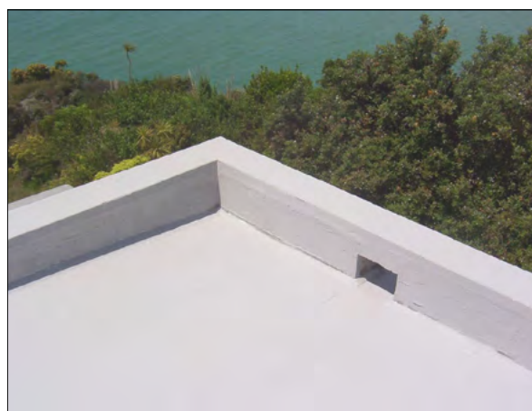
Detailing to parapet and scupper
