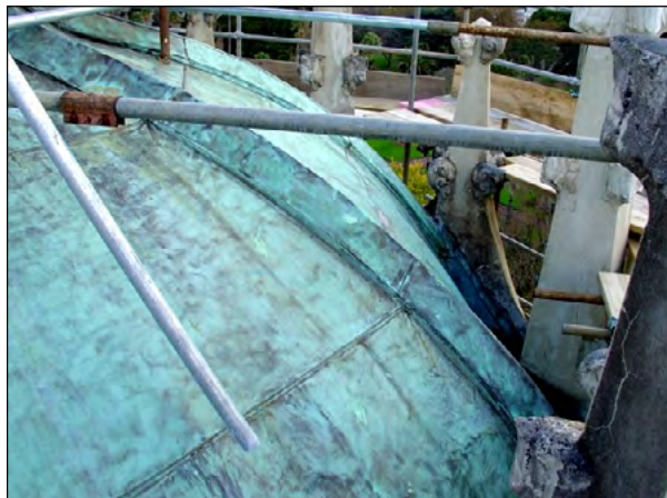
Original weathered copper roof
