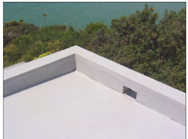
Detailing to parapet and scupper
