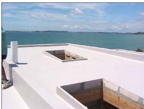
Dexx and fibreglass detailing around skylights
