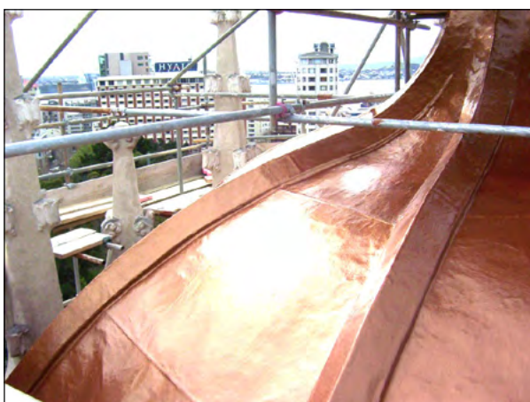
Copper DEXX Bodycoats with Fibreglass reinforcement
