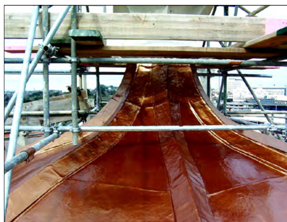
Chevaline Chemglaze protective clear finish applied
