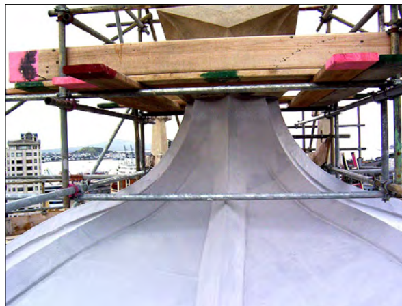
Chevaline DEXX base coat applied over copper
