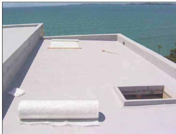
Fibreglass encapsulation into wet Dexx bodycoat
