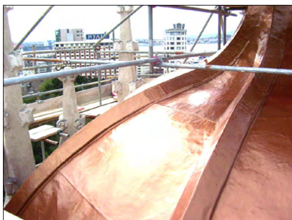
Copper DEXX Bodycoats with Fibreglass reinforcement
